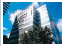
ATMC Taiwan Manufacturing Center
