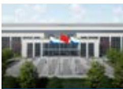
Electric Power Distribution Industry
